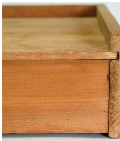
Machine-planed drawer bottom. With the introduction of planers in the late 19th century, drawer bottoms could be planed thin enough to fit into narrow grooves without the need for bevels or rabbets.
