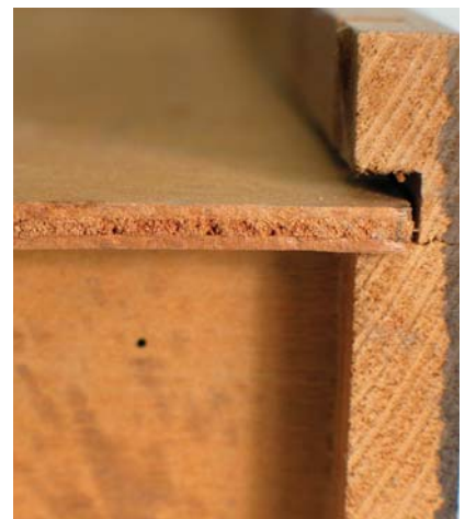
Plywood drawer bottom. By the 1910s manufactured plywood was available and it quickly replaced solid wood as the drawer bottom material of choice.
