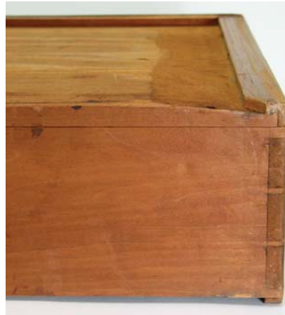
Handplaned drawer bottom. Drawer bottoms made before the machine age are typically thicker and are beveled on three edges to fit into narrow grooves cut into the drawer front and sides.
