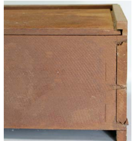
Rabbeted drawer bottom. Drawer bottoms made in the late 19th century after the introduction of band saws and large table saws are often rabbeted on three edges to fit narrow grooves cut into the drawer front and sides.
