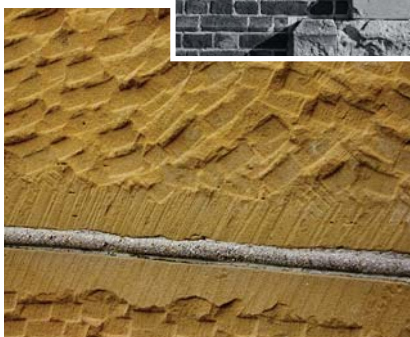
Texture. Beyond the rough patterns of nature, carving chisels can be employed to create an endless variety of textured patterns.
