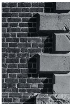
Shadow lines. A border consisting of small blocks with deep chamfers creates texture, the result of distinct shadow lines.
