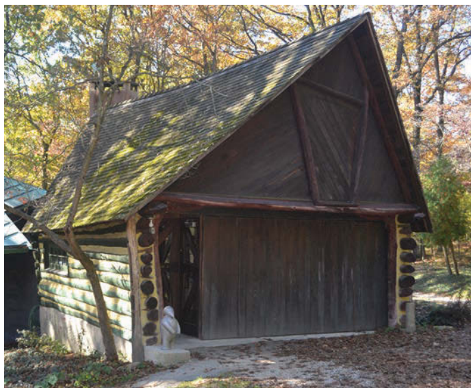
Flowing ridgeline. The visitor's center at the museum is housed in what was Esherick's garage. His desire to create a complete environment for himself led him to shift the axis of the ridgeline of this roof to create an asymmetrical appearance (right).
