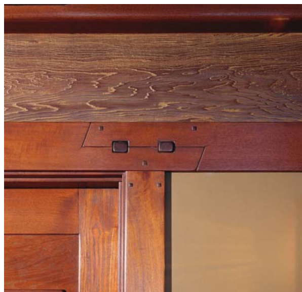
Simple solution. Unlike the redwood in the billiard room, the wire-brushed frieze in the upstairs foyer of the Blacker house had to be gently cleaned and waxed.
