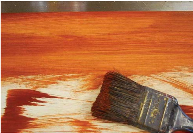
Grain. The bulk of the graining is applied with a very stiff, old brush to achieve a lined finish. Don't aim for straight strokes; variation adds a lifelike look.
