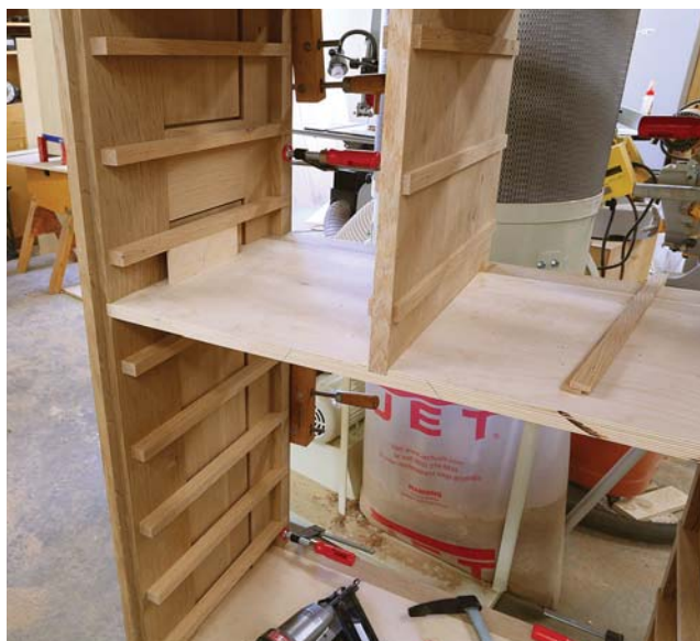
Drawer guides. The drawer guides are simply nailed in place to the case sides and center divider; on the sides, they are rabbeted around the trim strip at the front. Note the spacer that holds the guides level as they're nailed.
