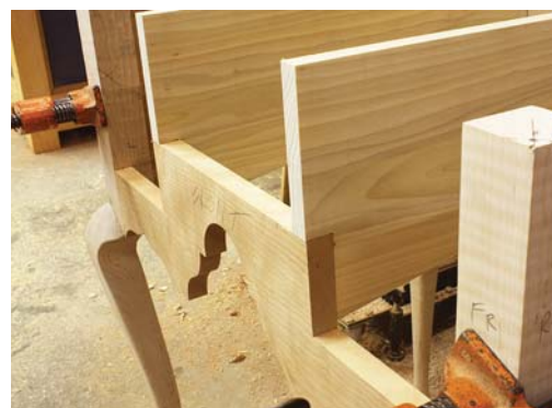
Piggyback. Drawer dividers ride on the front apron and sit in dados at the back. That's easy work.
