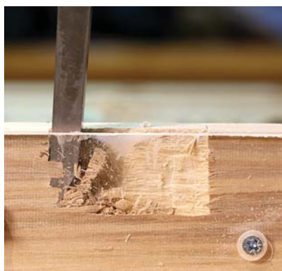
At the end. After removing the bulk of the waste, chop straight down at the ends. It's OK if the end cuts are not perfect.
