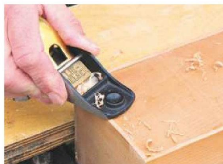
15 With the box held upside down, plane the panel edges flush with the base
