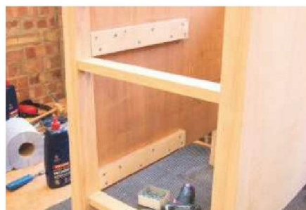
17 Cut, drill and fit plywood side spacers as shown to carry the drawer runners
