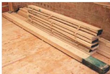
1 Stack the raw timber using stick spacers and allow it to acclimatise for two weeks
