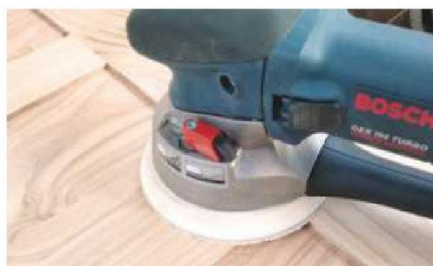
25 Sand the assembled back smooth and screw it into its rebate
