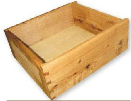
12 The 6mm ply drawer bottom, meanwhile, was housed in slots cut in the front and sides
