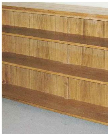
13 The bookcase has a vertical support mid-way along the shelf length as belt and braces for support for heavyweight reading matter
