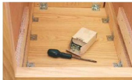
46 Fix the two pedestals to the desktop using metal shrinkage brackets
