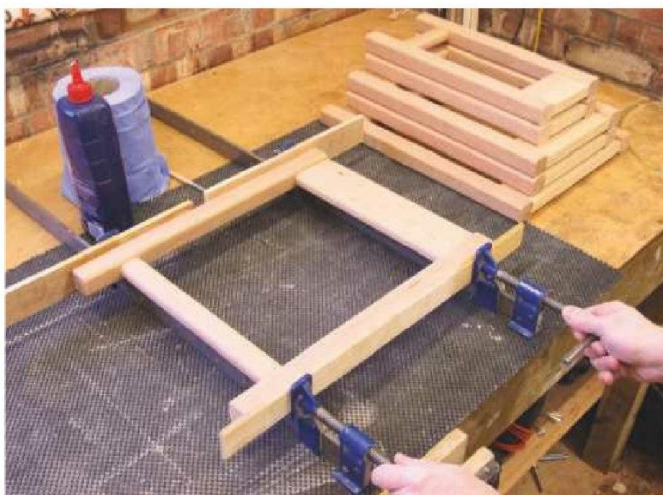
7 Glue up each frame in stages, starting with a pair of legs and the side rails
