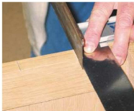
21 Mark the hinge positions and cut the ends of the recesses to depth with a tronsaw.
