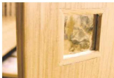
26 The stained glass inlays were retained by four mitred pieces of glazing bead
