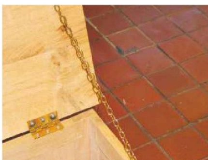
24 Fit the eyes and chain to one (or both) sides of the chest to stop the top opening too far.
