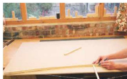
41 Mark the different arc shapes on the desktop template with a string bow
