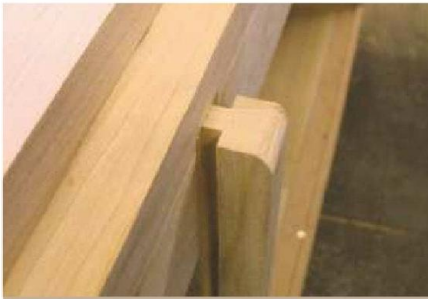
21 The central divider has a groove at each side into which the two back panels slide
