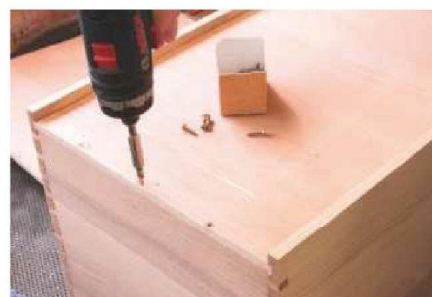
29 Glue each drawer base in place and screw the front and rear edges
