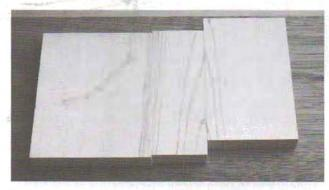
5-14. Saw cuts in straight and angled grain areas of a board. Notice the degree of offset at the ends of the boards required to match the grain when the cut is made in an area with angled grain lines.
