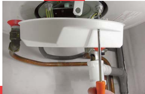
2 - Retirez le capot de protection.
